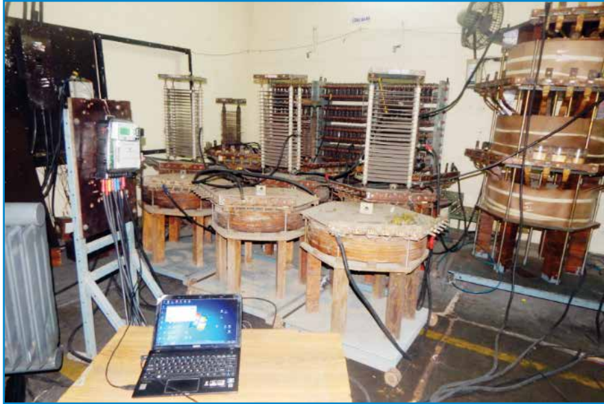
Testing of 240V, 5-30A single Phase two wire UC2 Prepaid energy Meter
