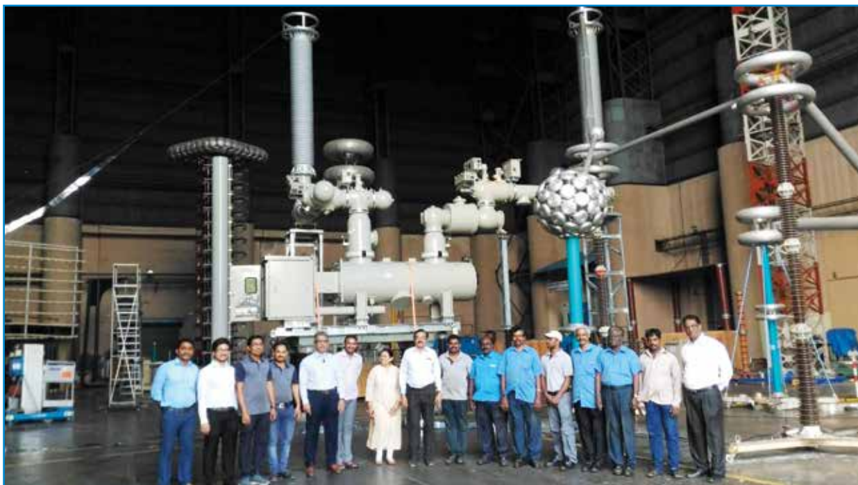
Dielectric and RIV tests were carried out as per IEC 62271-203 on 245 kV SF6 Gas insulated switchgear and 400kV SF6 Gas insulated switchgear
