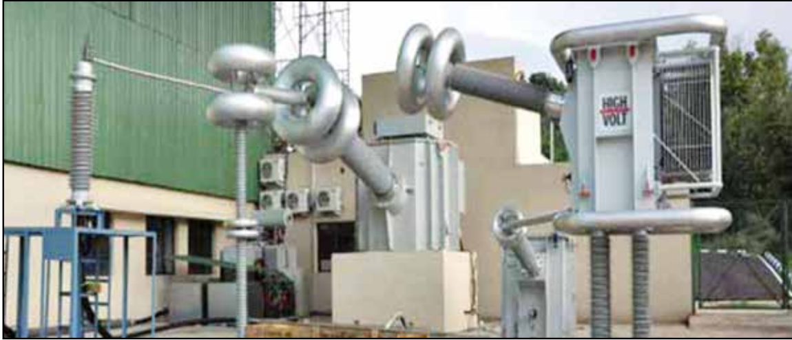
600kV, 4200 kVA Outdoor Transformer
