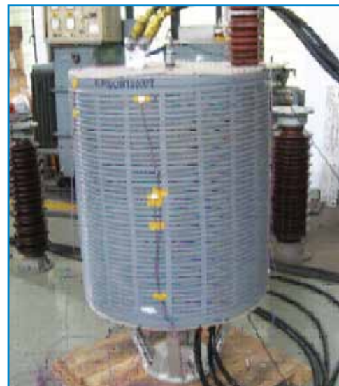
0.2 mH, 1250A, Line trap undergoing temperature rise test
