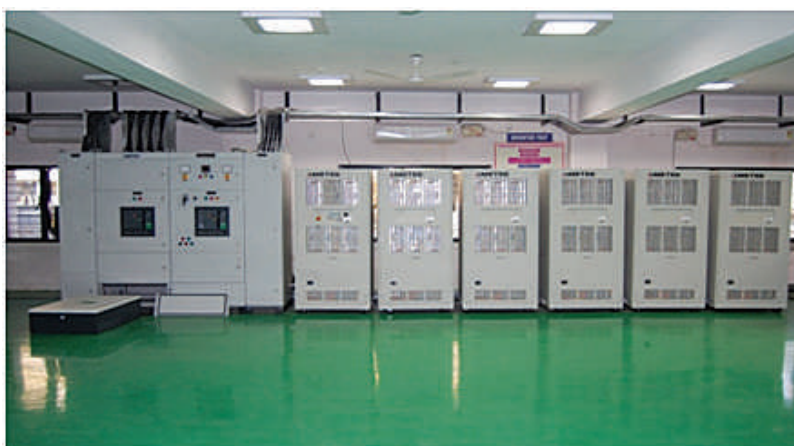
Testing of inverters
