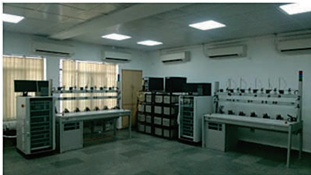
Energy Meter Test Laboratory at RTL-CPRI, Noida
