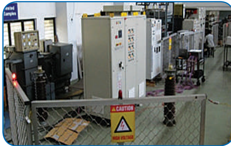
A view of the 3 \Phi , 500 kvar, 440 V, LV APFC panel undergoing tests in the Capacitors Division
