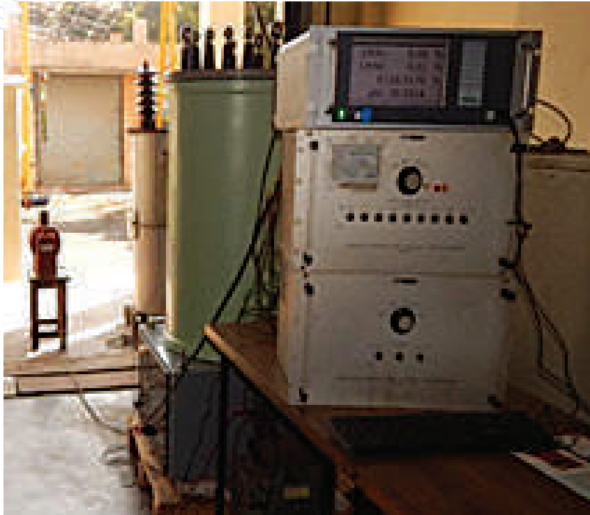
33000 V/ \sqrt{3} / 110 V/ \sqrt{3} resin cast Potential Transformer during Accuracy test
