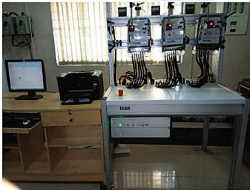
Photograph of 3 phase 4 Wire a.c. Static direct connected Watthour Smart Meter Class 1 is under metrological test
