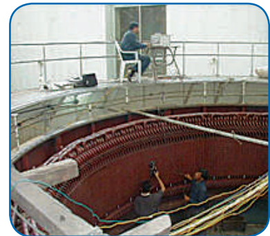
ELCID Test on Hydro Generator
