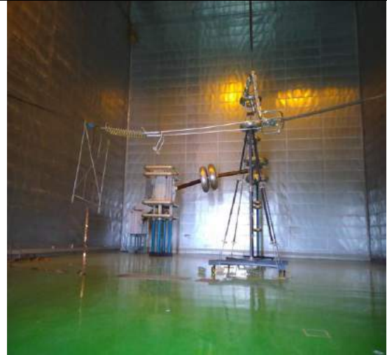
132 kV Double Tension Insulator String
