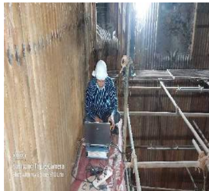
Corrosion mapping of boiler water wall tubes in progress
