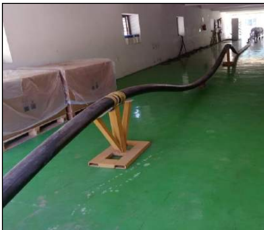
Cable laid inside the open tunnel with Zigzag pattern
