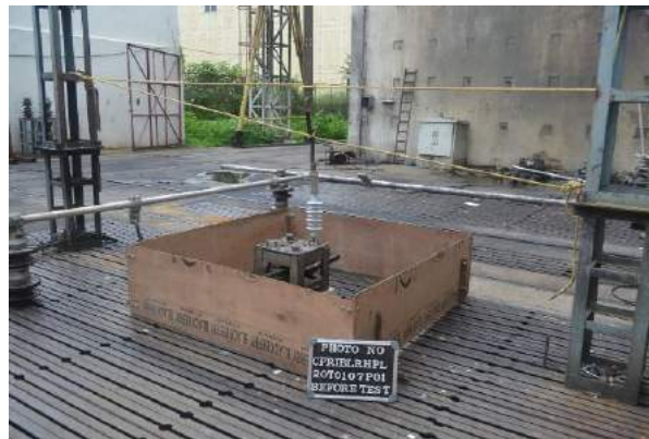
Short circuit tests on 22kV of Lightning Arresters
