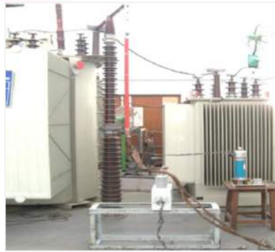
Arrangement for Over Voltage Test on 120kvar, 3.8kV, Fuseless HV capacitor
