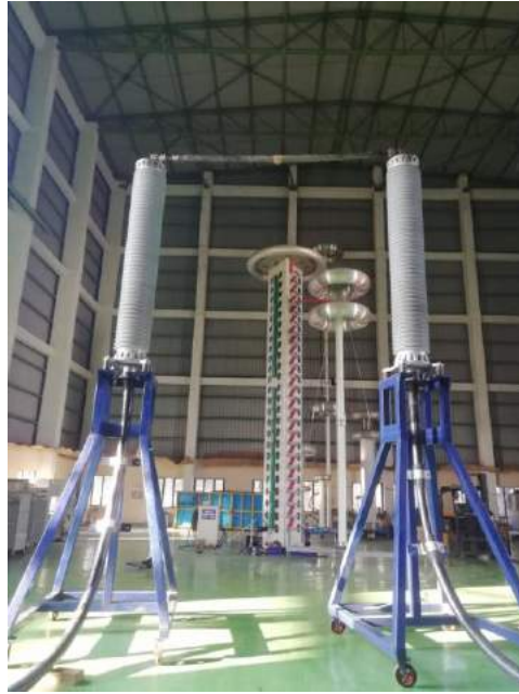
Lightning Impulse Voltage test set up
