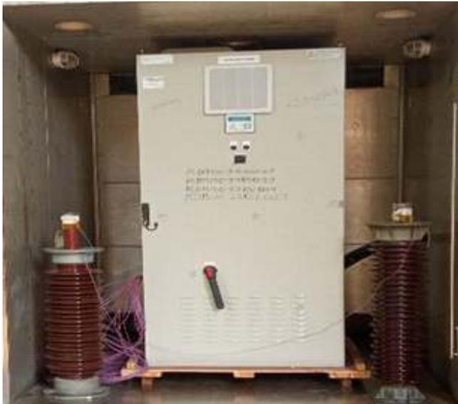
**Compact APFC Panel of rating 550kVAR, 440V, 3 Phase, 50 Hz**
