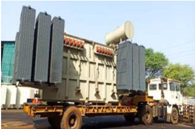
**18 MVA, 33/0.69-0.69-0.69-0.69kV, Five Winding Aluminum Wound, Inverter duty Transformer**
