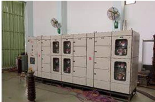
A view of the tested 3Ø, 440V, 800 kvar LV APFC Panel
