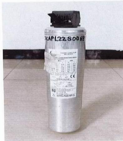
**A view of the tested 30kvar, 440V, 3Ø, MPP Type LV Shunt Capacitor**
