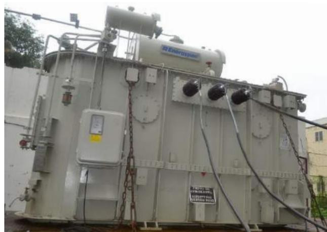
**Dynamic ability to withstand short circuit test on 16/20MVA, 33/11.3 kV three-phase Transformer**
