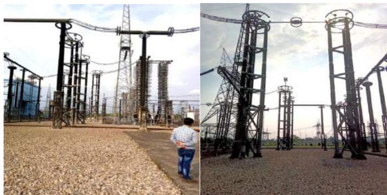
**DC Electric field measurement at  $\pm 800$  kV, HVDC Terminal Station of M/s. Power Grid Corporation of India Ltd., Biswanath Charali**
